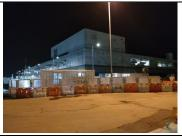
Control of night-time lighting by hooding and minimisation of night working period (CM7)
